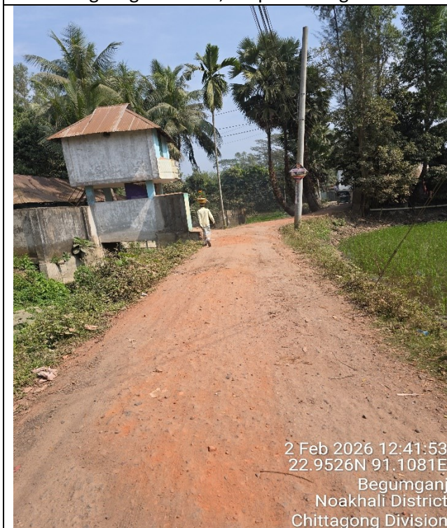
UT-95: Type of Road: Existing BC/Earthen road. Existing length: 290 m; Proposed length: 290 m.
