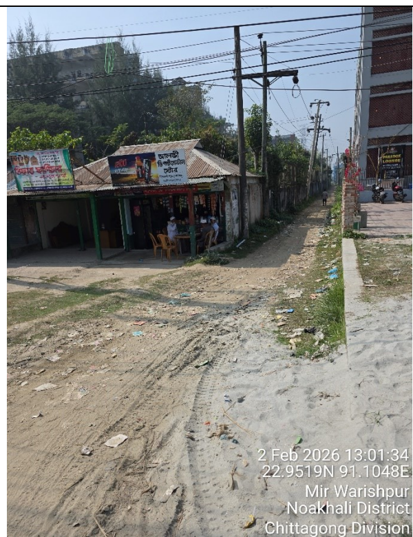
UT-27: Type of Road: Earthen road. Existing length:400 m; Proposed length:400 m.
